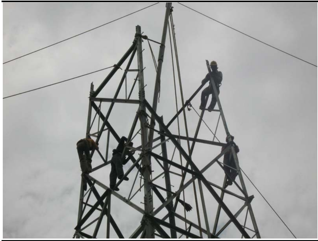
Figure 1.11 Erection of tower
