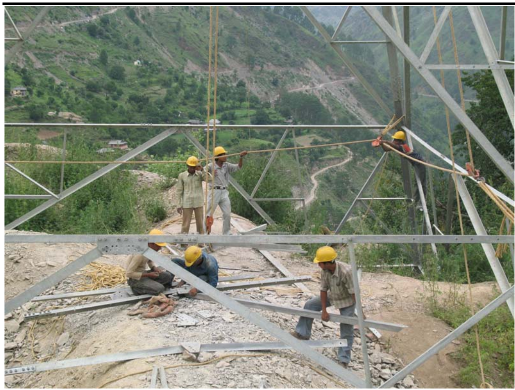
Figure 1.10 Joining the tower lattice
