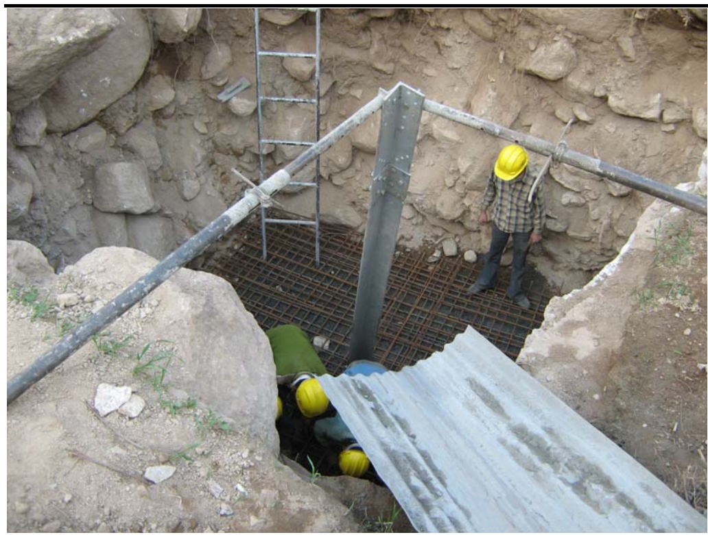
Figure 1.6 Foundation pit for tower
