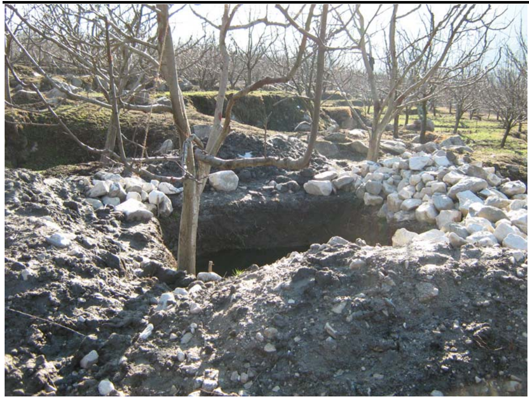
Figure 1.3 Foundation pits for Tower
