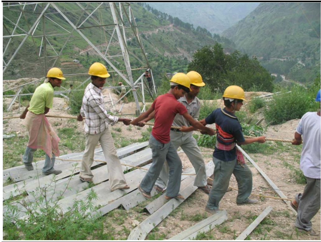
Figure 1.13 Stringing Process
